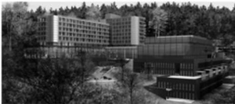
Lufthansa Training &amp; Conference Center in Seeheim
